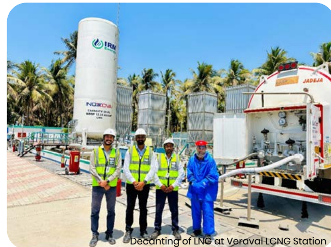
Decanting of LNG at Veraval LCNG Station
